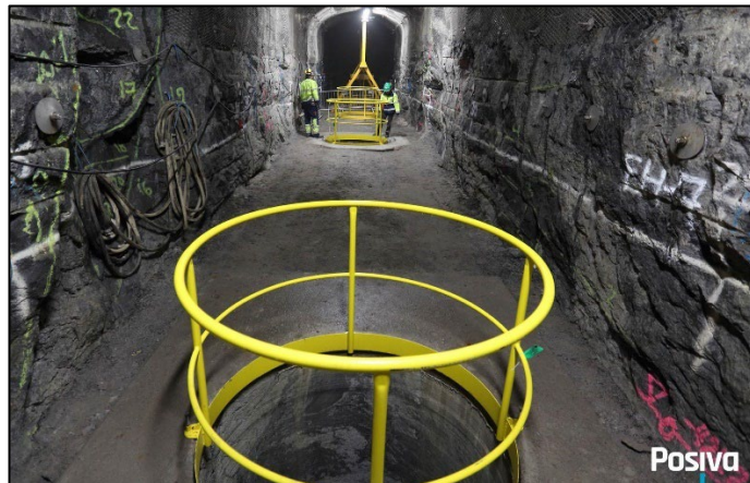
Figur 5.2 Deponeringsbrønner i det geologiske deponiet i Onkalo i Finland. ( https://www.posiva.fi/en/index.html )
